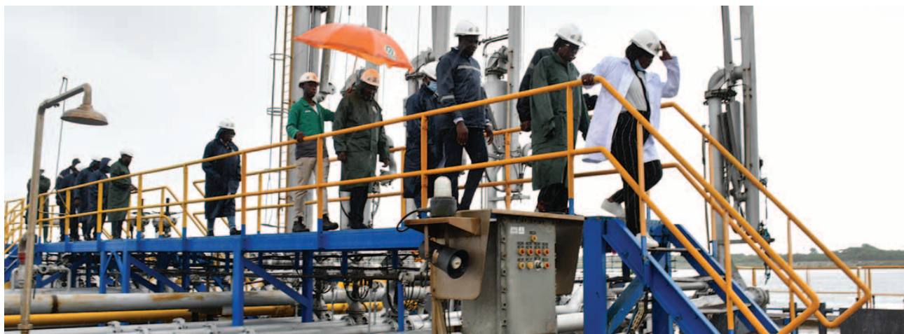
Visite des installations des appontements de PETROCI Visit of PETROCI's wharf facilities
